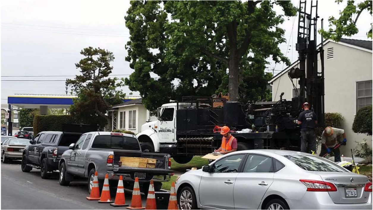
Photo 1- Boring 3 drilling, April 24, 2015, 1749 Malcolm Avenue
