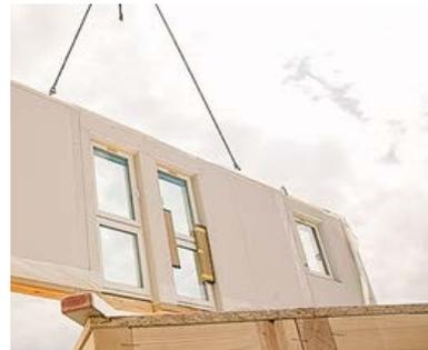
Built in a factory and arranged on site with huge cranes; this is a high quality and efficient building process that comes with a large price tag.
