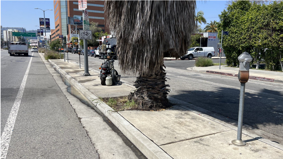
PHOTOS FROM CITY OF LOS ANGELES BUREAU OF SANITATION AND ENVIRONMENT
