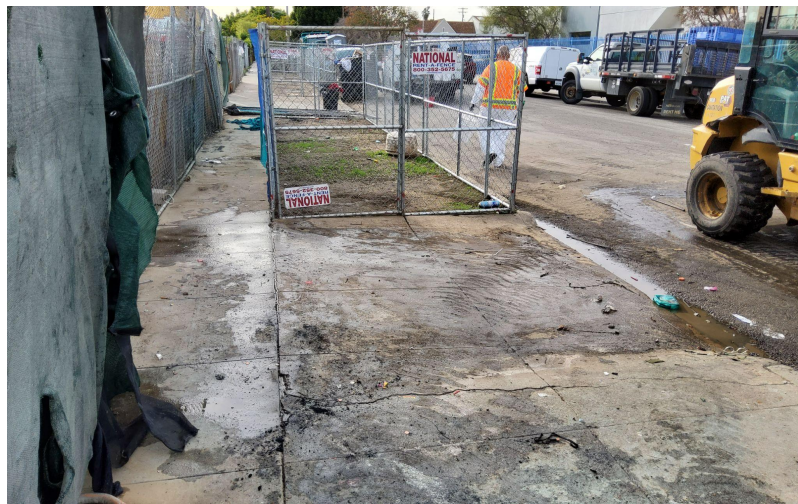
PHOTOS FROM CITY OF LOS ANGELES BUREAU OF SANITATION AND ENVIRONMENT
